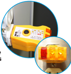
Traditional receptacle test indicates circuit is good.
