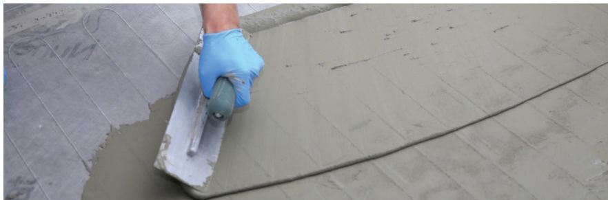
FIGURE 2.21: Install tile/stone flooring
