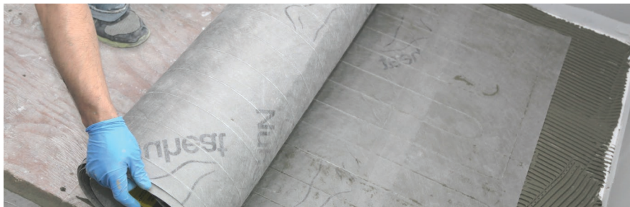
FIGURE 2.13: Place mat onto fresh thinset
