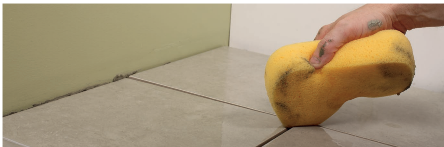
FIGURE 2.23: Clean grout lines
