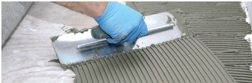
FIGURE 2.12: Spread thinset onto subfloor
